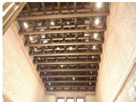
The original structure (left photo), presumably of wrought iron, is visually light with additional decorative features of dubious structural value. Chipperfield's version (right photo) is a series of ponderous, dark-coloured Vierendeel girders, a structural form unknown at the time of the museum's conception.
