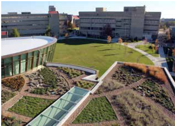
Green roofs reduce stormwater impacts on Narragansett Bay, moderate temperatures on hot days, and add value to views from taller buildings
